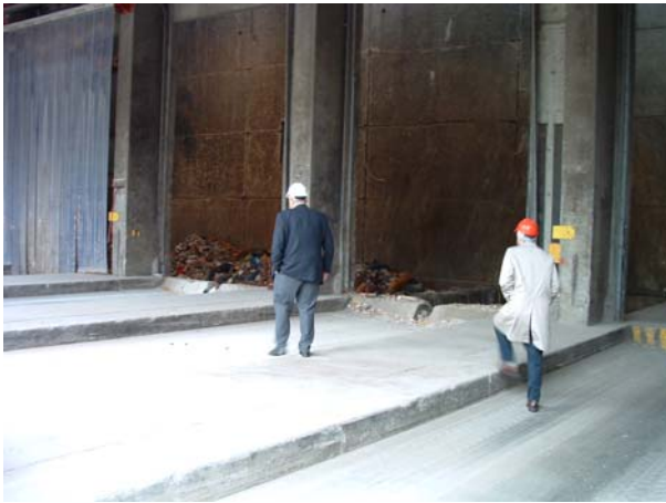
MSW is dumped into the waste bunkers in the tipping hall.
