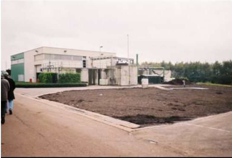
Wastewater treatment plant for landfill leachate and excess liquid from digestion
