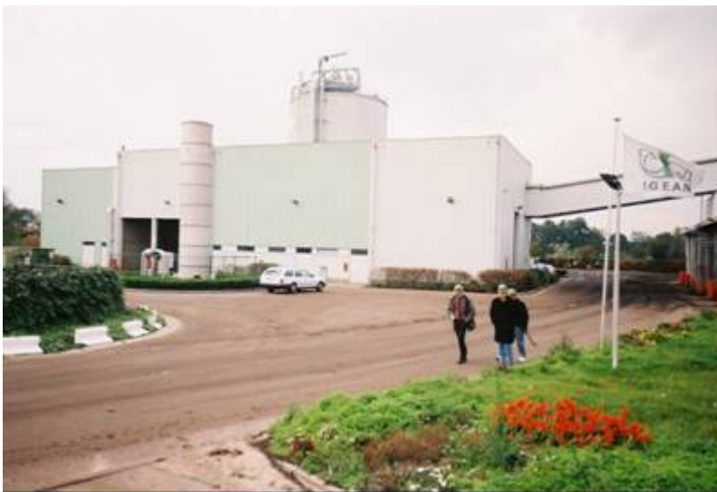
Brecht II, entrance; emergency flare in foreground, preprocessing building behind it, digester in background
