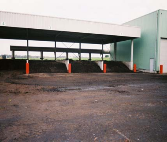
Front side of biofilter
