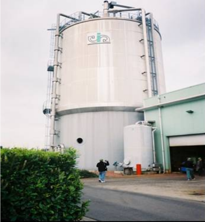
Dranco digester with feeding pipes along the sides; the bottom third contains the conical bottom of the digester
